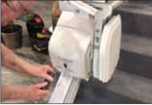
Attach bottom cover of drive train .
