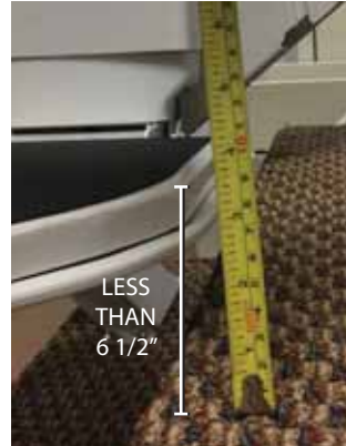
MEASURE AT TOP & BOTTOM LANDINGS TOP OF FOOTREST TO FLOOR HAS TO BE LESS THAN 6 1/2"
