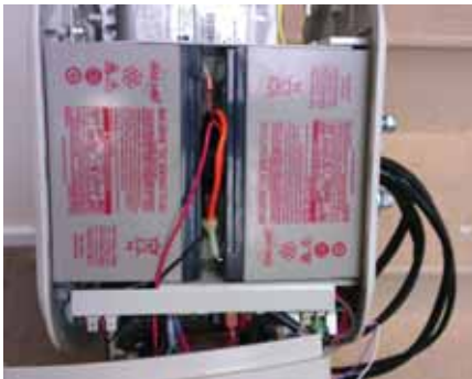
BATTERIES ROTATED BACK IN PLACE
